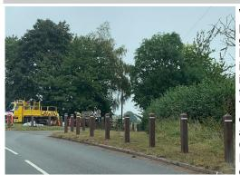
With a view to protecting the grass verge at Low Habberley, it was decided to install bollards at this location. The bollards are of а type approved by County Council Highways to collapse in the
